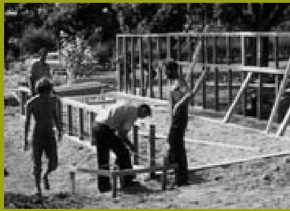
BUILDING THE GREENHOUSE
