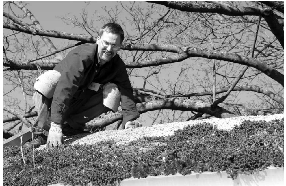
Demonstration Garden volunteer Will Polk replaces growth media on the peak of our greenhouse's green roof. Photos by Grace Seidel
